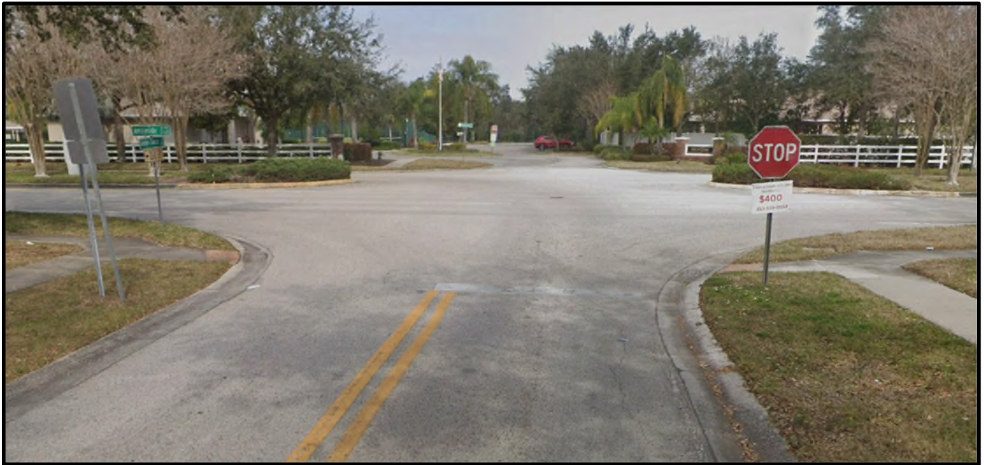
Figure 4: Golden Silence Dr South Approach looking North
