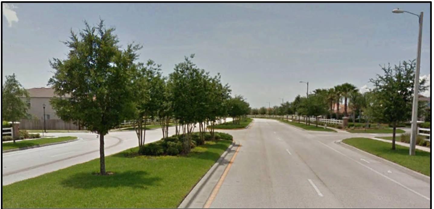
Figure 3: Ambleside Blvd West Approach Looking East
